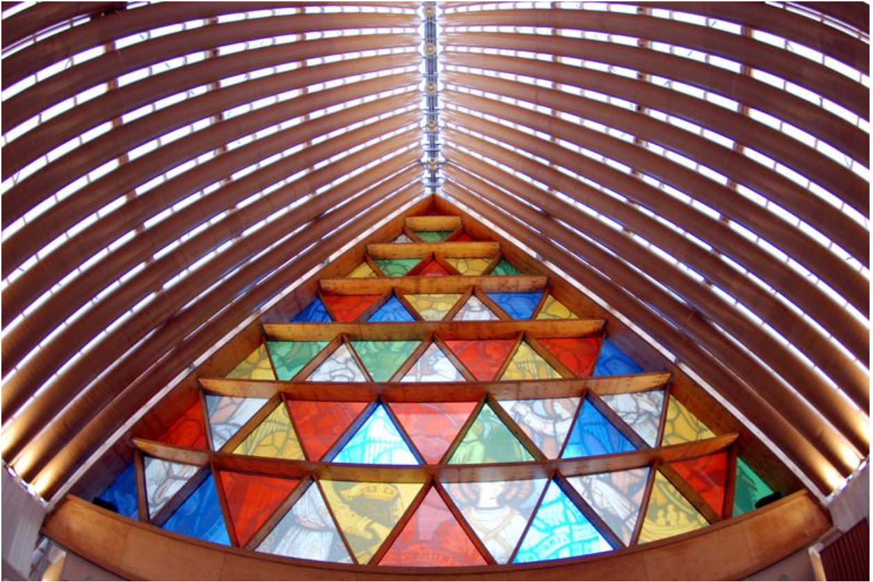
Transitional Cathedral, Christchurch, New Zealand. The world's only cathedral made substantially of cardboard
